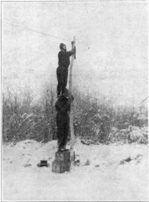
FIXING ONE OF THE INSULATORS OF THE MAIN TELEPHONE LINE TO THE OLD FORT RAE.
