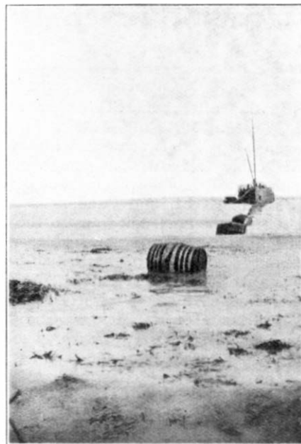
FIG. 4.—FLOATING THE CABLE ASHORE AT ST. MARGARET'S BAY.
