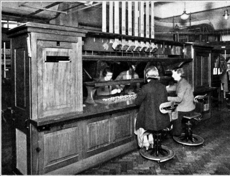
FIG. 4.—P.D.P. IN INLAND TRUNK EXCHANGE CONVERTED FROM MIX AND GENEST TO MCGREGOR TERMINALS.
