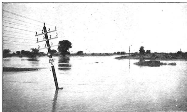
FIG. 12.—LINES DAMAGED BY FLOODS.
