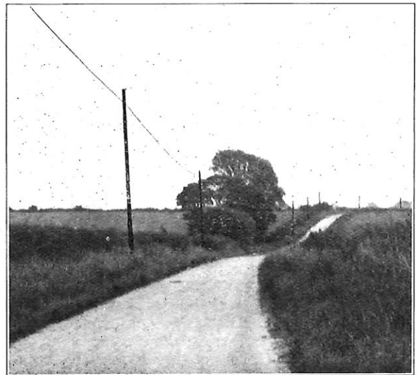
FIG. 8.—A SECTION OF CONTINUOUSLY SUSPENDED AERIAL CABLE.
