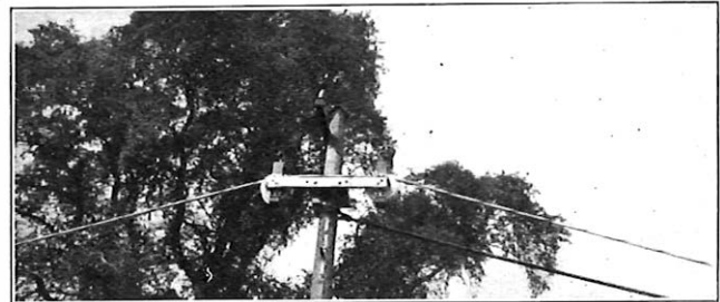
FIG. 3.—CABLE SHEAVES SECURED TO POLE.
