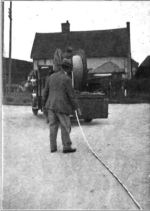
FIG. 6.—PAYING OUT CABLE FROM LORRY.
