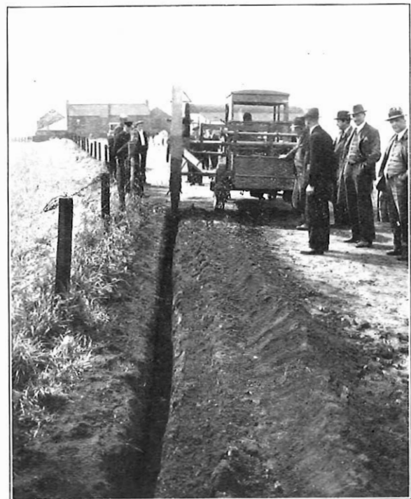
FIG. 2.—TRENCH EXCAVATOR IN ACTION.
