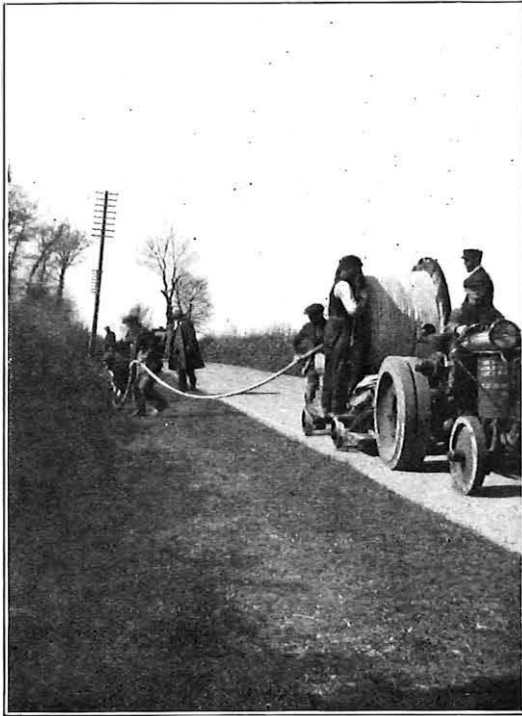
FIG. 4.—LIFTING CABLE INTO POSITION.
