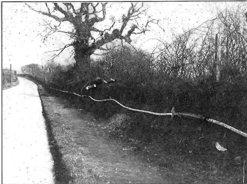
FIG. 5.—CAST IRON COUPLING OVER JOINT
