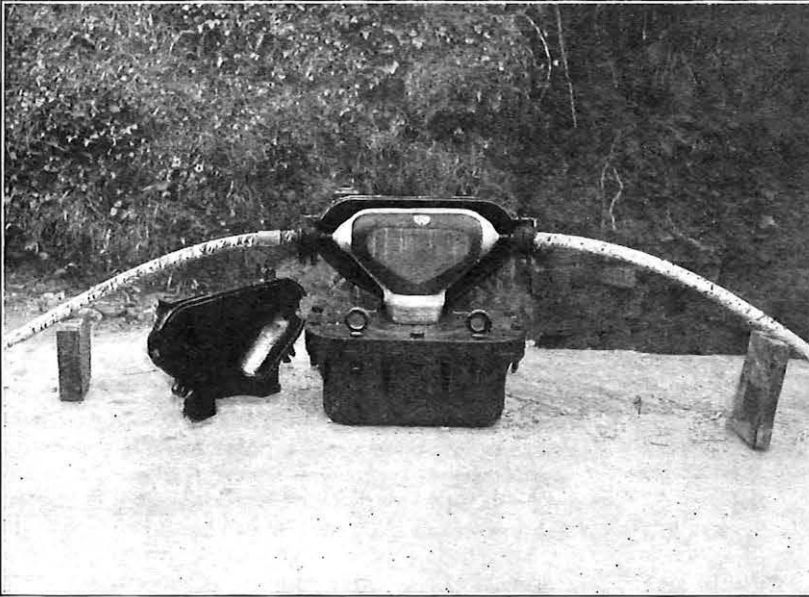
FIG. 2.—BURIED LOADING POT.
