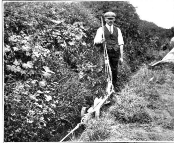
Fig. 11.—Small Mole Drainer in action in ploughed furrow. Note cable entering joint hole.
