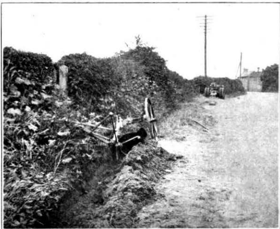
Fig. 9.—Plough drawn by winch with Furrow 10"—12" deep.
