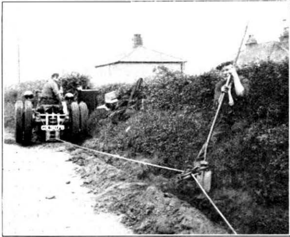
Fig. 7.—Portable anchor and pulley block used where steel hawser turns a sharp corner.
