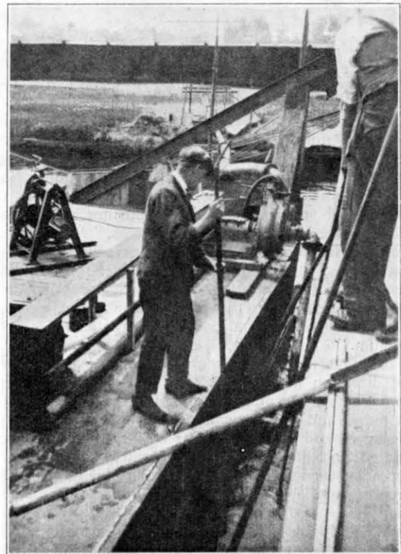
FIG. 1.—MOTOR PUMP MOUNTED ON BARGE.
