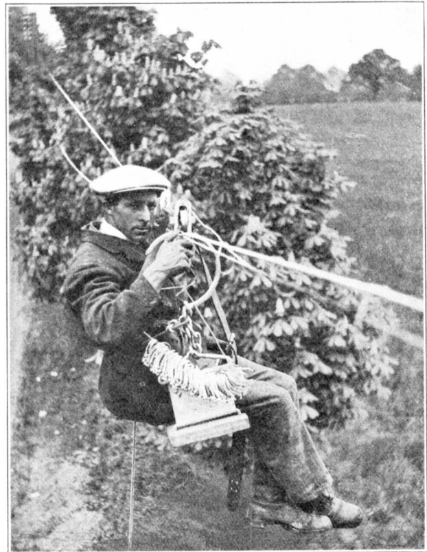
FIG. 4.—WORKMAN FITTING RINGS.
