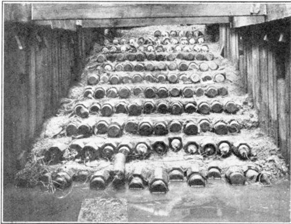
FIG. 6.—PARTLY CONSTRUCTED 126-WAY DUCT.
