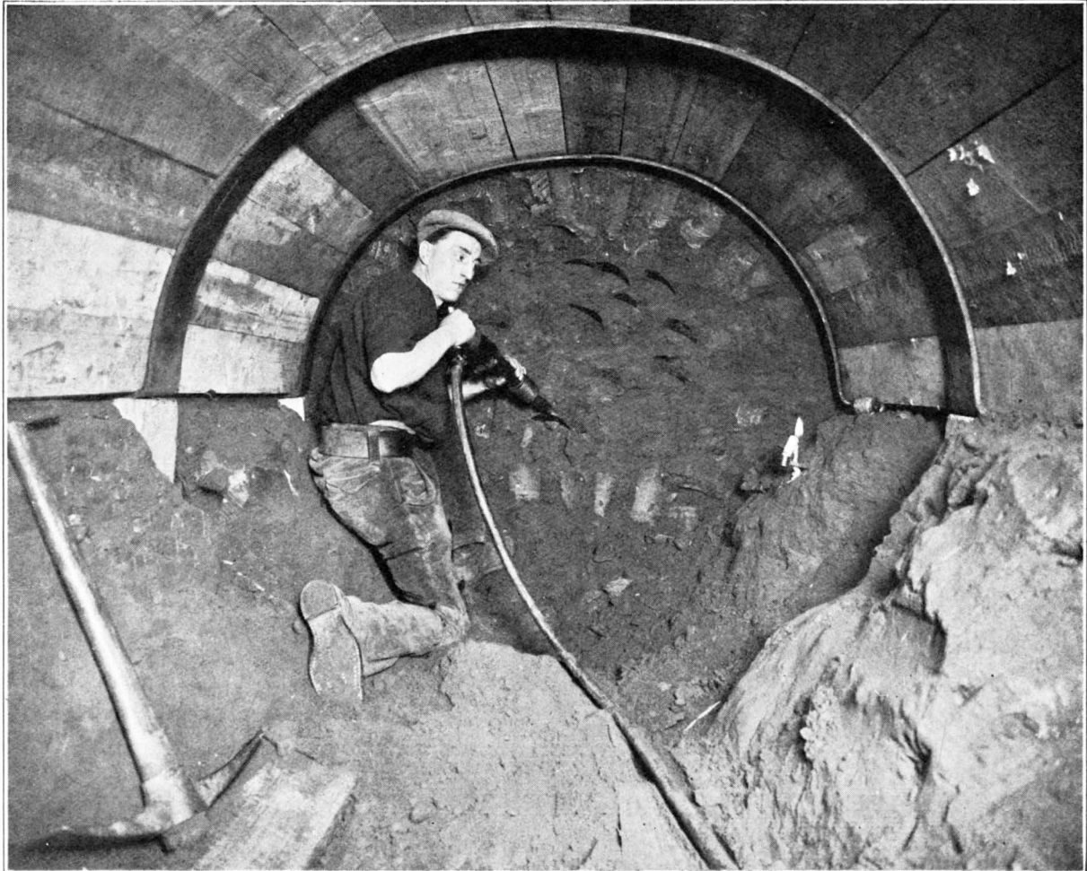
FIG. 14.—TUNNEL UNDER MANCHESTER-ROCHDALE CANAL: EXCAVATING.
