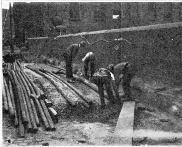
FIG. 3.—VICTORIA BRIDGE. LAYING STEEL PIPES.
