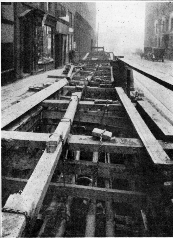
FIG. 11.—TRENCH FOR 70-WAY DUCT-LINE, BLACKFRIARS STREET, SALFORD.
