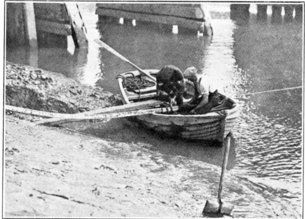
FIG. 4.—LASHING CABLE TO BOAT.
