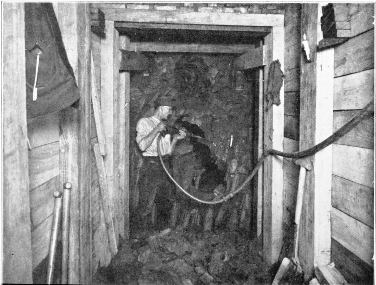
FIG. 7.—EXCAVATION OF A TUNNEL.
