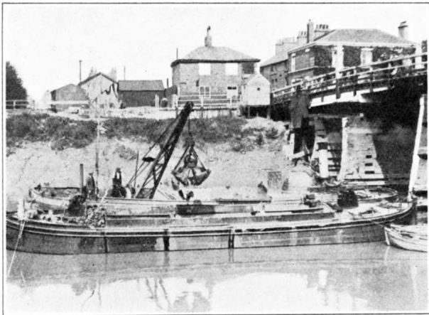
FIG. 2.—DREDGER CUTTING CABLE TRENCH.
