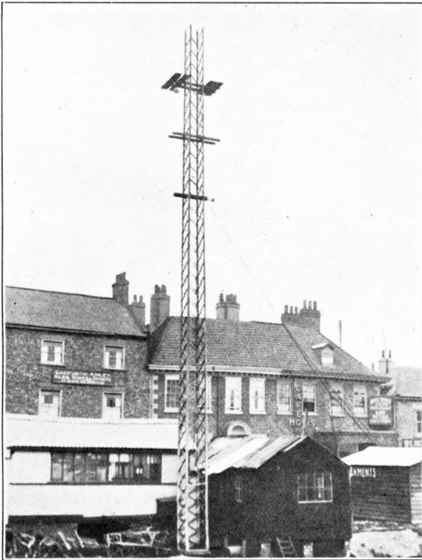
FIG. 1.—STAGING AND OXYACETYLENE APPARATUS.
