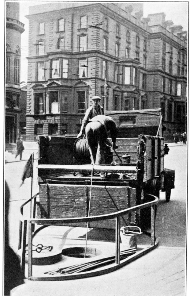
FIG. 8.—STEEL HAWSER AFTER LEAVING THE CAPSTAN BEING COILED ON HAWSER WINDER.
