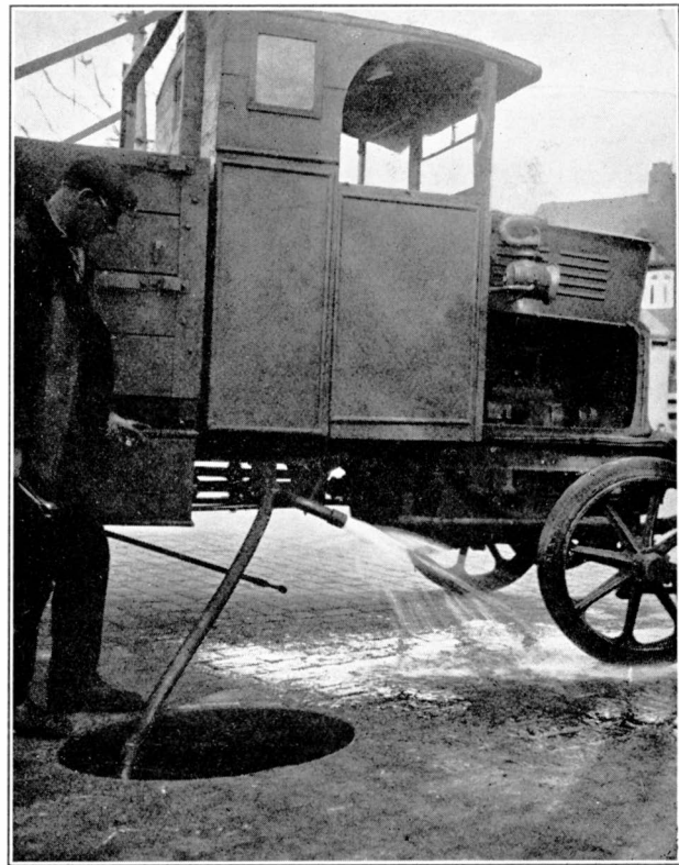
FIG. 9.—PLUNGER PUMP IN OPERATION.
