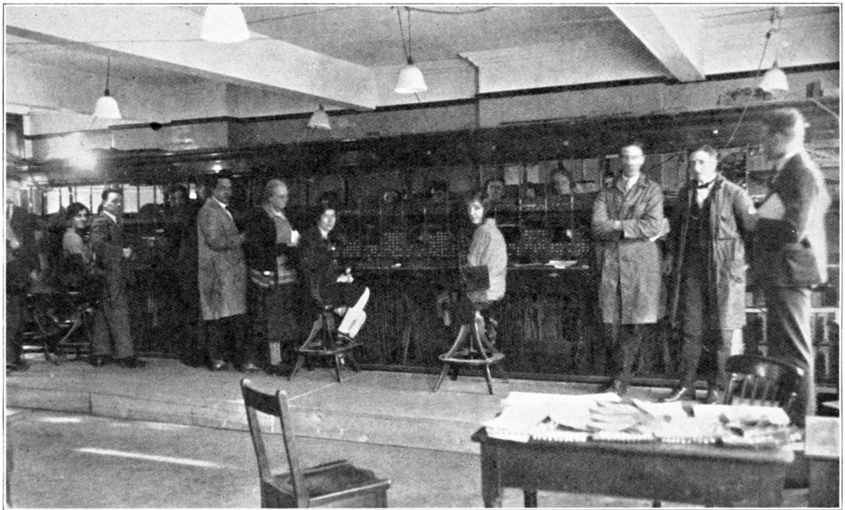
FIG. 1.—EMERGENCY MANUAL SWITCHBOARD, SHOWING STATE OF RECONSTRUCTION ON 4TH MARCH, 1929.
