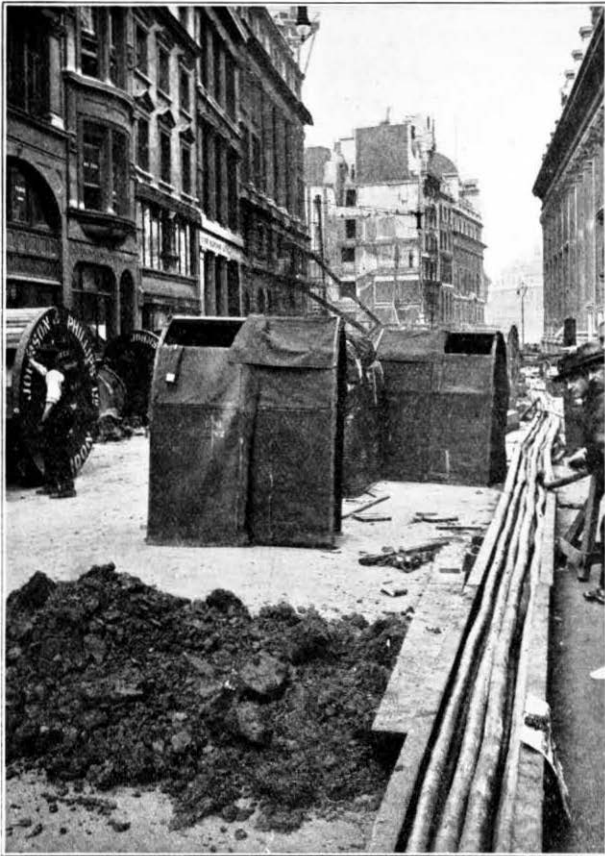
FIG. 3.—OPERATIONS IN CORNHILL SHOWING CABLES IN TROUGHING.
