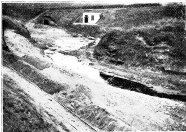
FIG. 4.—CABLE HUT AT AUDRECELLES.
