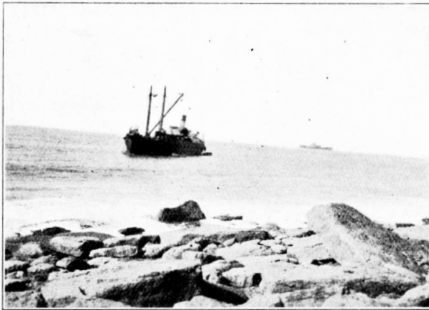
FIG. 1.—THE "DRUDGE" GOING IN WITH SHORE END.
