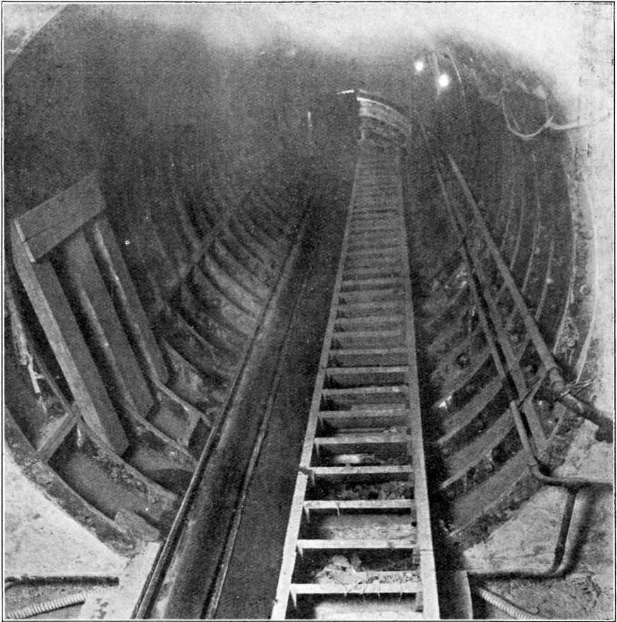
FIG. 11.—LOOKING UP SLOPING TUNNEL.
