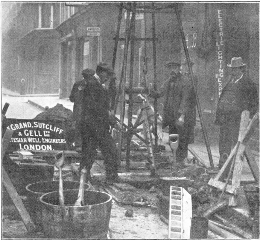
FIG. 4.—BORING IN PROGRESS.
