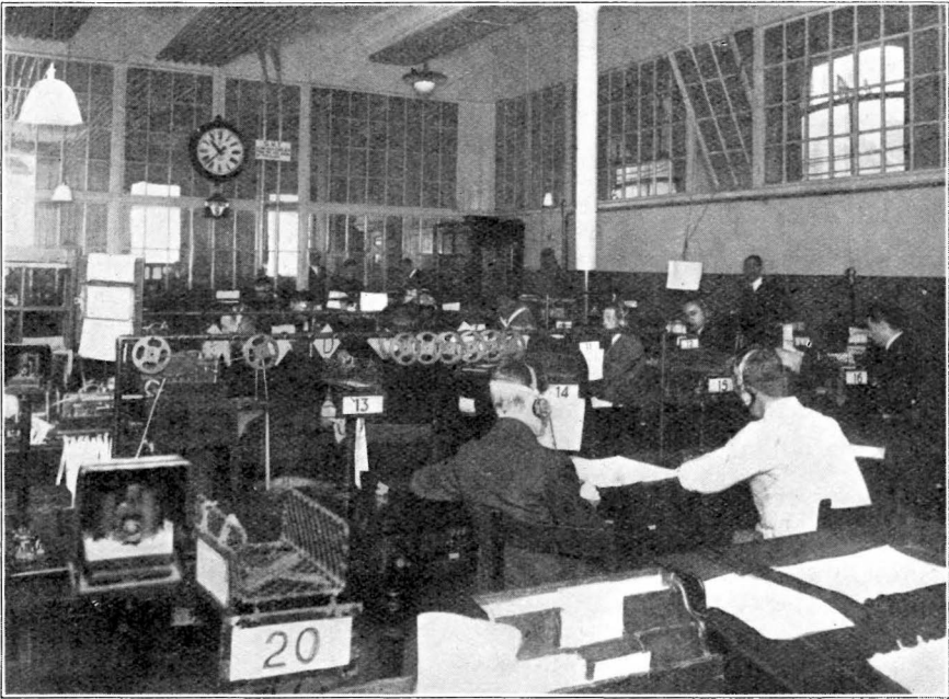
FIG. 1.—CENTRAL RADIO OFFICE, G.P.O. WEST.
