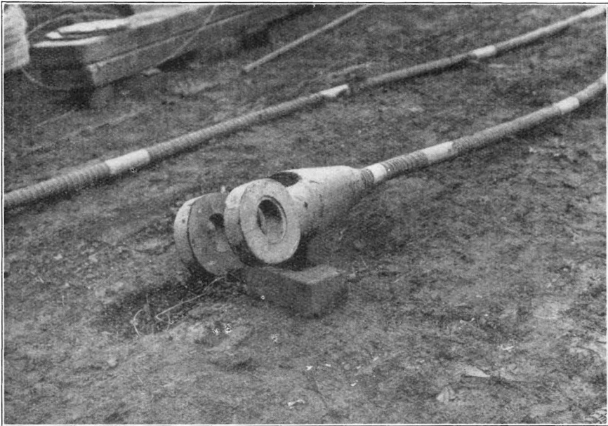
FIG. 3.—SOCKETS AT END OF STAY ROPE.
