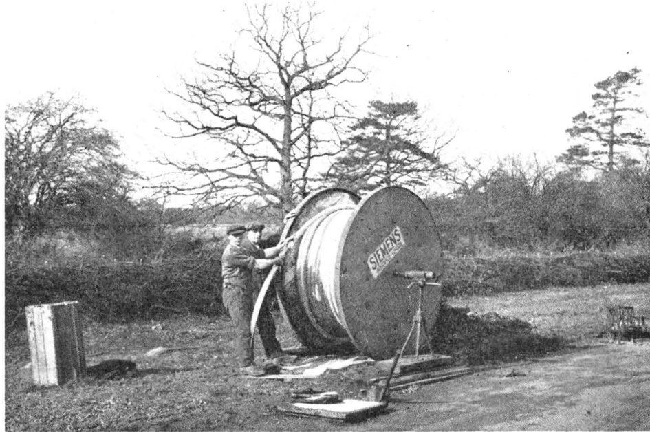
Drawing in Trunk Telephone Cable along a country road.
