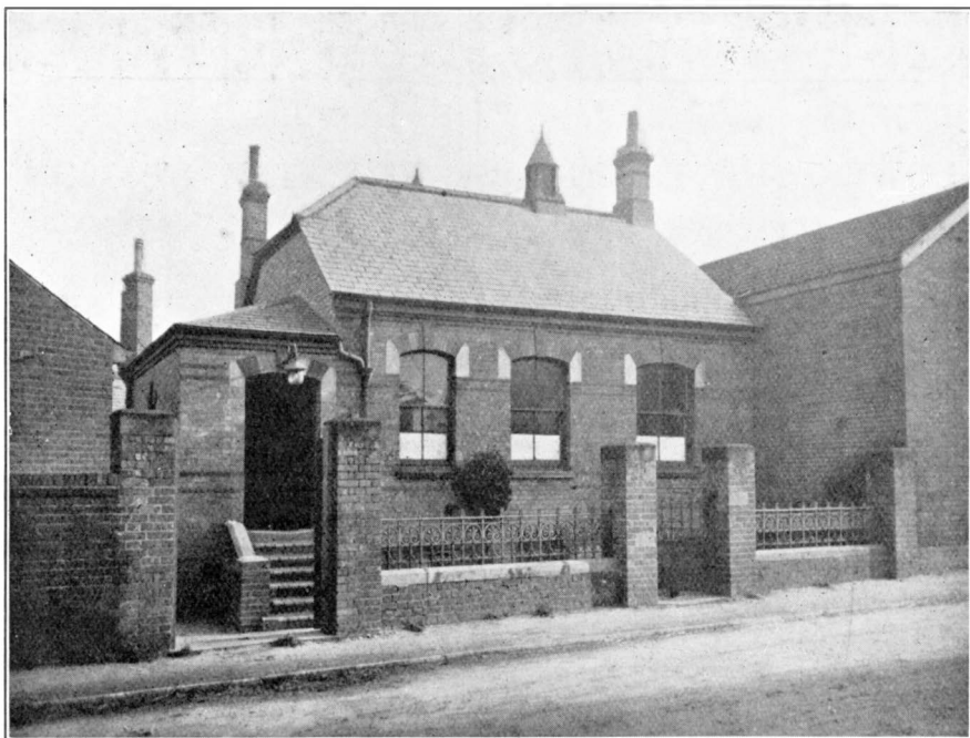
FIG. 1.—LOWESTOFT REPEATER OFFICE.
