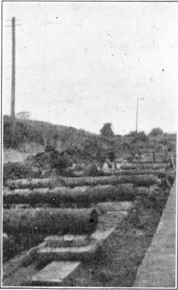
FIG. 2. TIMBER BAULKS ACROSS TRENCH SHOWING PACKING UNDER ENDS TO OBTAIN HEADROOM.
