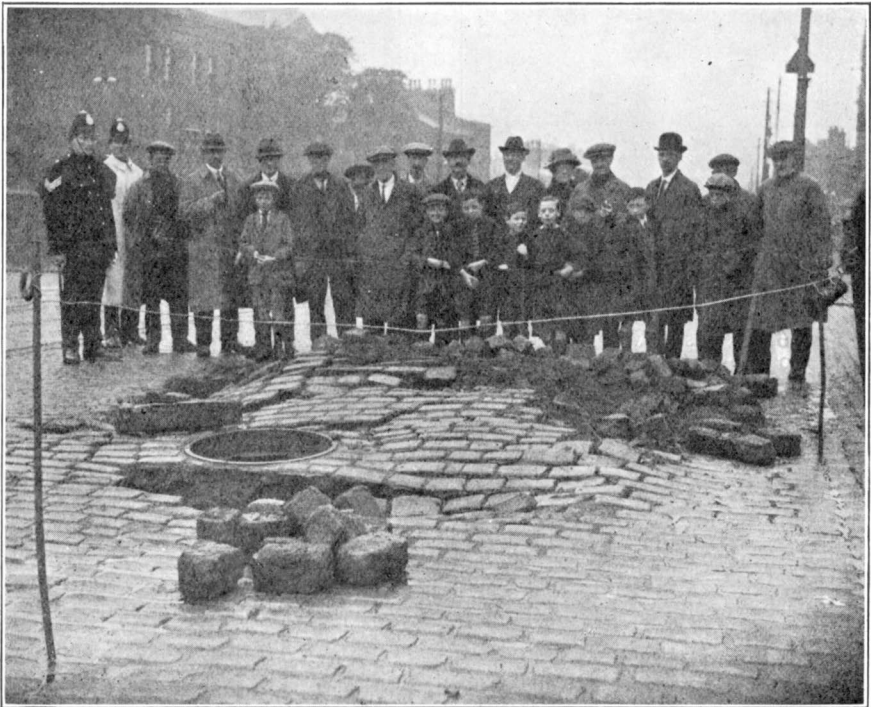
FIG. 1. ROADWAY ABOVE MANHOLE ROOF.
