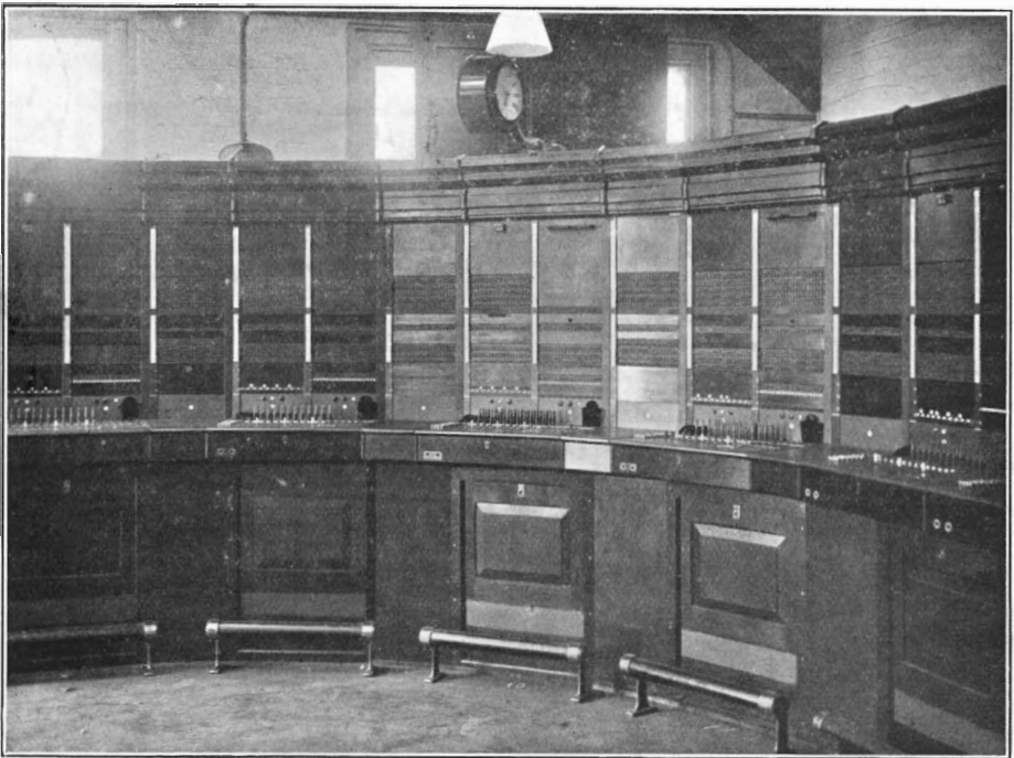
FIG. 2.—VIEW SHOWING MULTIPLE IN ANGLE SECTION.
