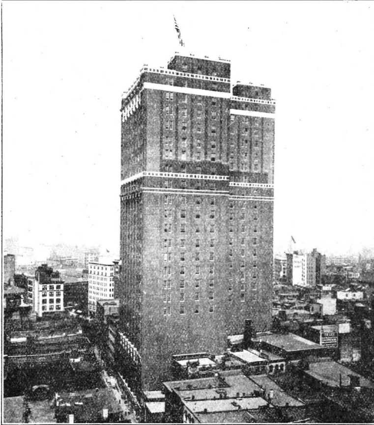
FIG. 3.—WALKER-LISPENARD TELEPHONE BUILDING, NEW YORK.
