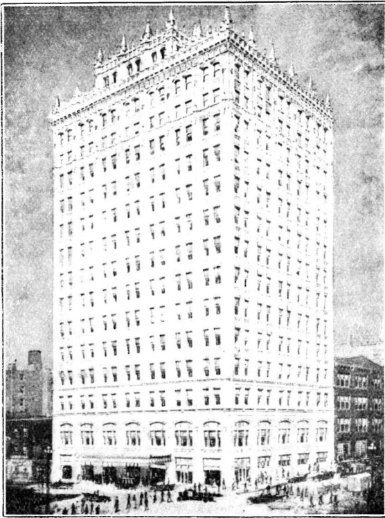
FIG. 4.—MAIN TELEPHONE BUILDING, KANSAS CITY.
