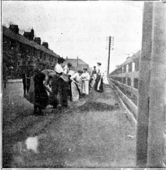
I.—DIGGING TRENCH, MIDDLESBROUGH.
