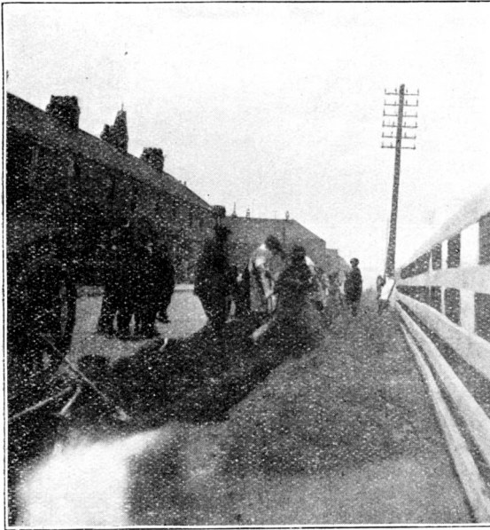
3.—LOWERING PIPES (3 LENGTHS) INTO TRENCH.
