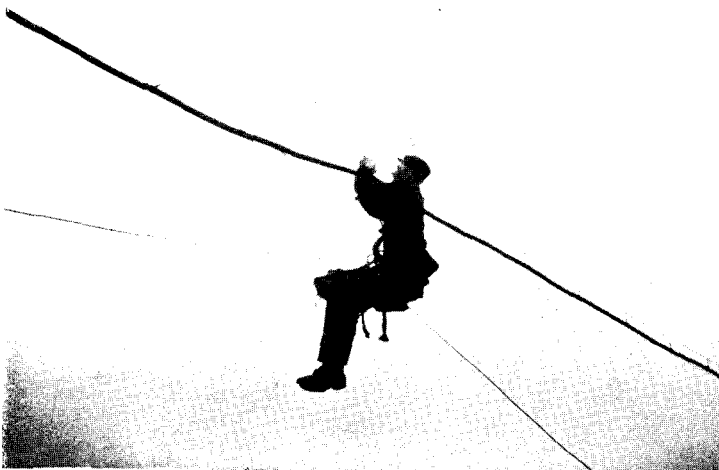
FIG. 4.—LONDON: CLERKENWELL, RENEWING CABLE SUSPENDERS AND SLINGS.
