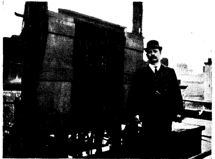
FIG. 5.—LONDON: COTHALL AVENUE JUNCTION BOX.
