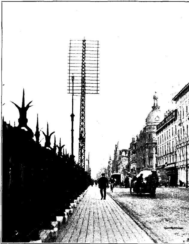
FIG. 4.—LATTICE-WORK GROUND POLE AT ANTWERP.
