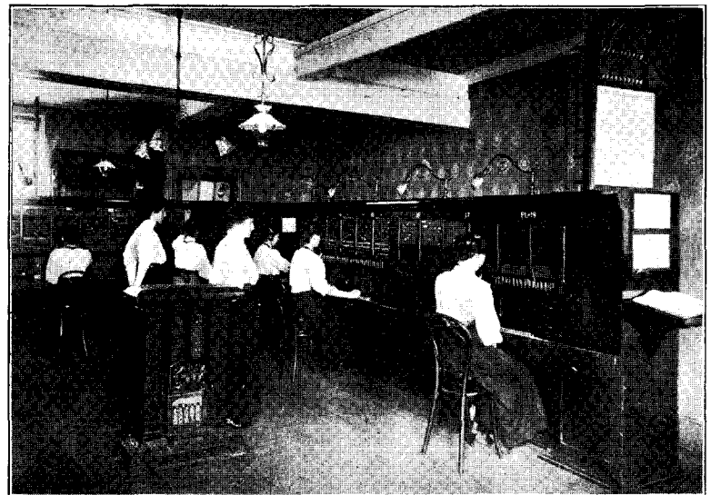
FIG. 5.—A CORNER OF BOURNEMOUTH SWITCHROOM.
