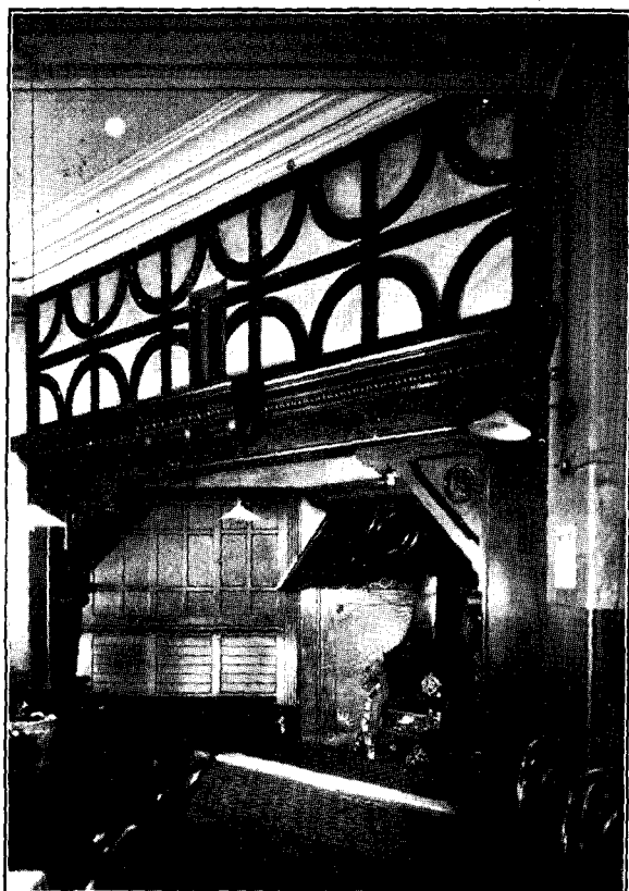
THE FIREPLACE IN THE OPERATORS' DINING ROOM, OLD GERRARD EXCHANGE.
