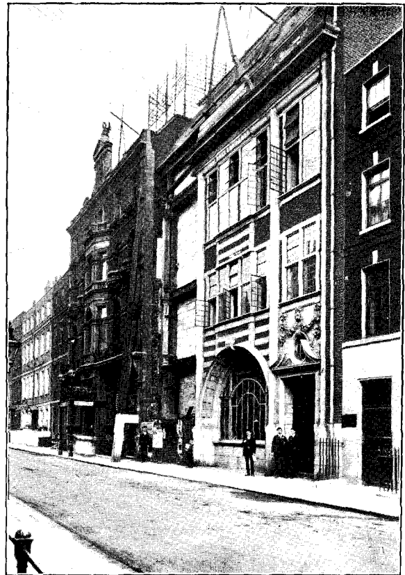
VIEW SHOWING OLD AND NEW BUILDINGS.
