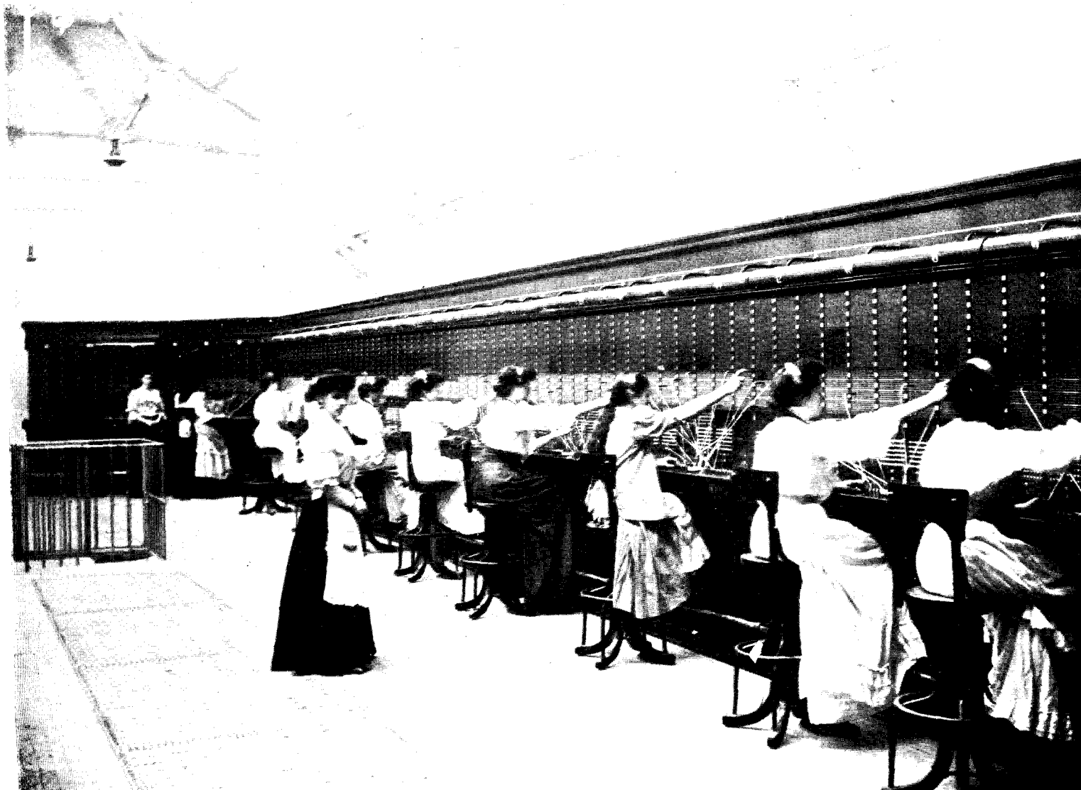
NEW "LIBERTAD" COMMON BATTERY EXCHANGE, BUENOS AIRES.
