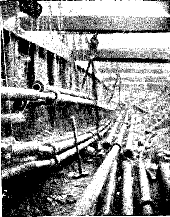
FIG. 4.—DUCTS PARTLY IN NEW POSITION.
