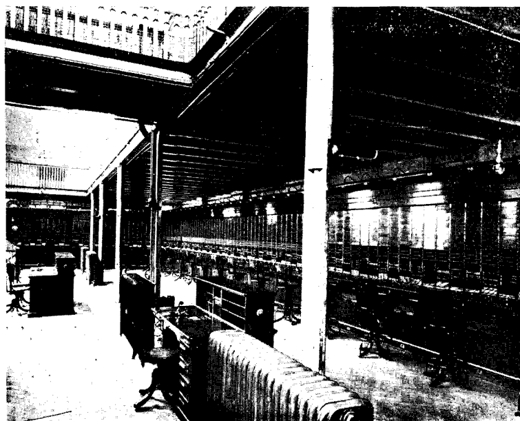
Hop Exchange, General View.
