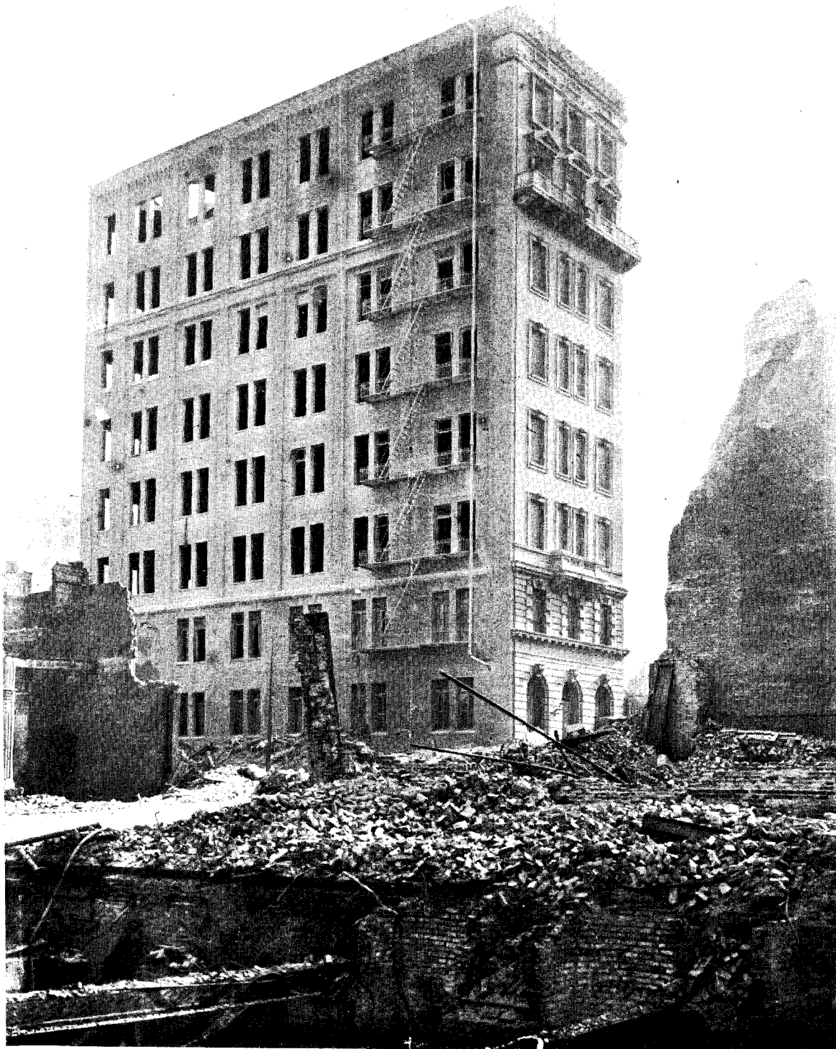
MAIN EXCHANGE BUILDING, SAN FRANCISCO, CALIFORNIA
