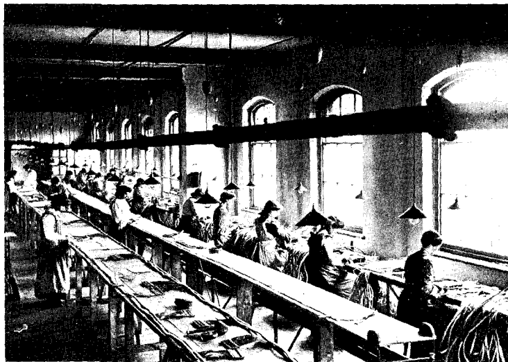
FIG. 8.—Showing measuring off, lacing, soldering, and examination processes in operation in Cable Shop.
