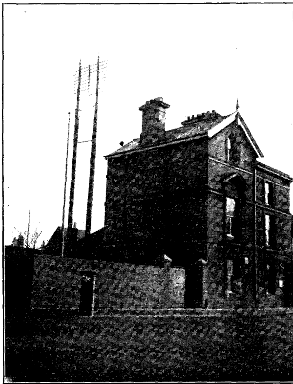
NEW GRIMSBY EXCHANGE BUILDING.
