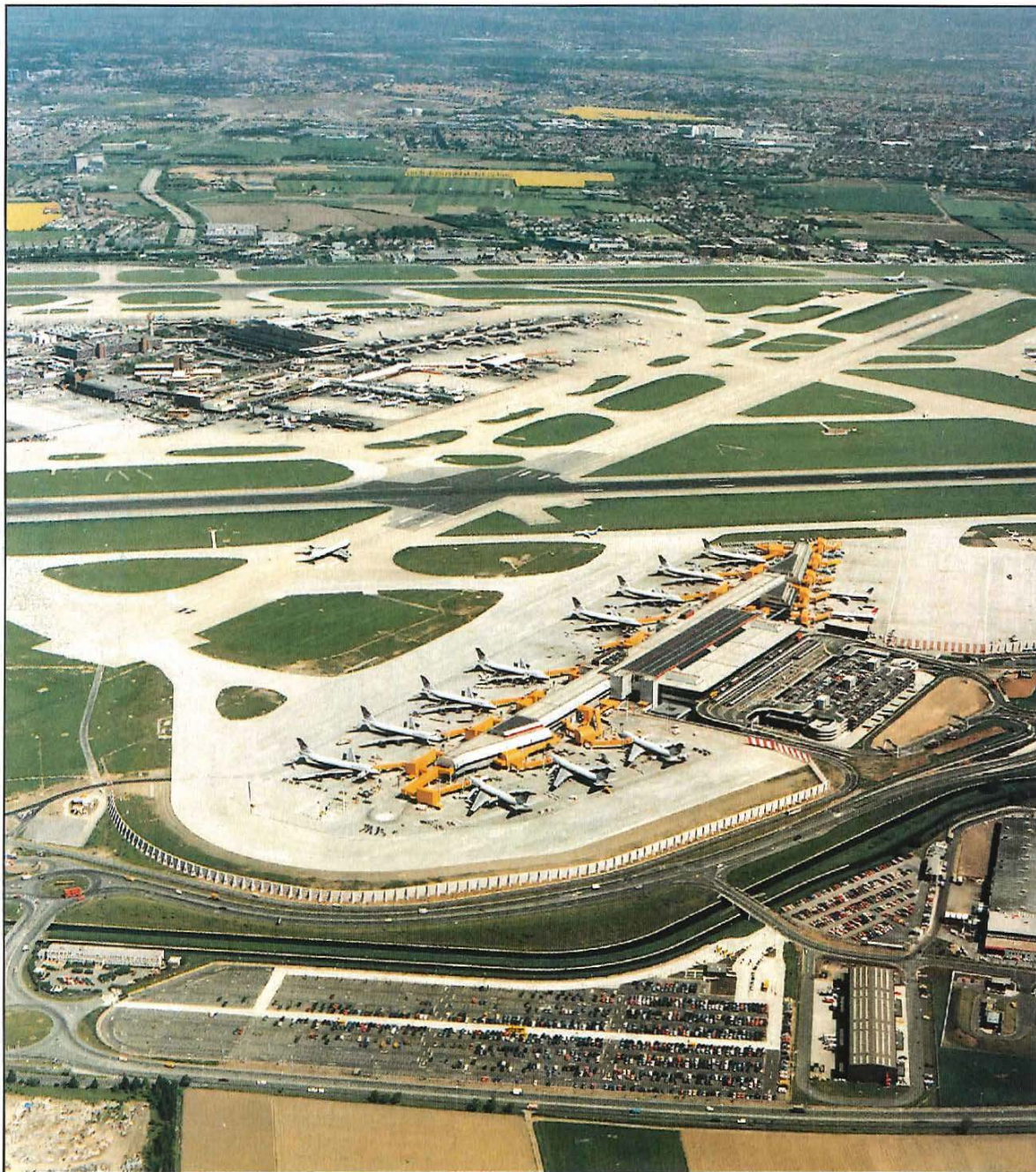
Heathrow Airport. Along with Gatwick and Manchester Airports it is served by ACP90 which provides air cargo processing facilities for imports and exports, and by DEPS which handles customs functions.
