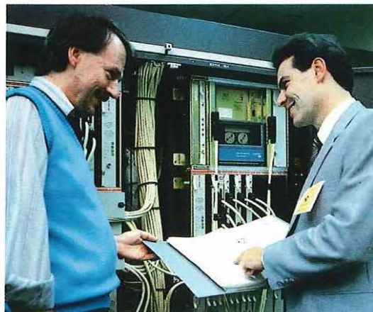
Installing exchange equipment at a customer's premises.
