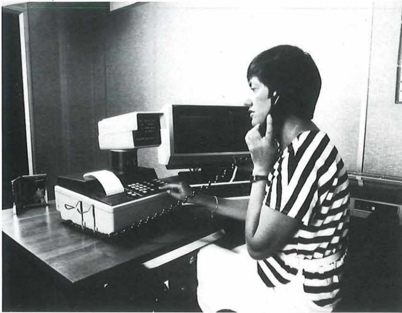
An operator takes an alarm call at the central control unit.
