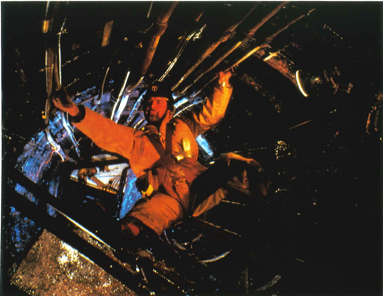
Installing optical fibre cables under the Hull river
