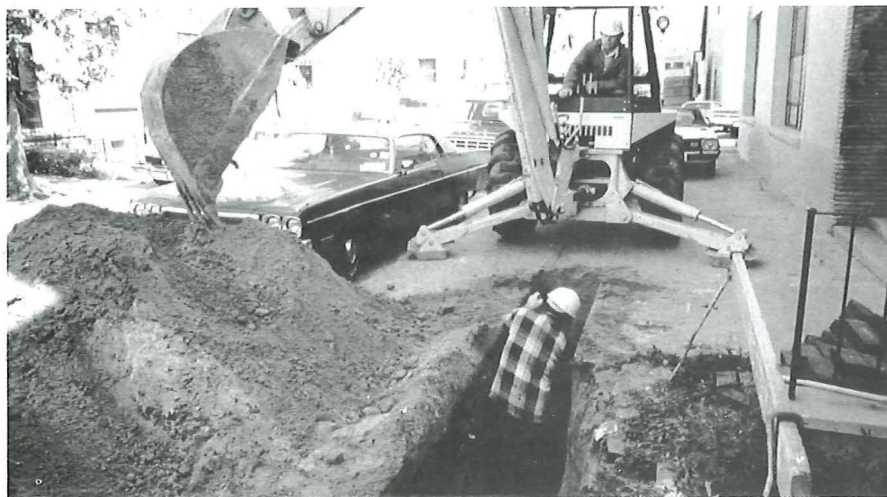
A Toronto construction crew install new optical fibre cable at Yorkville.
