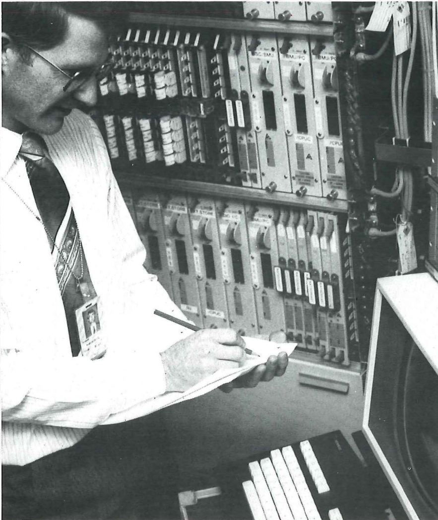
Executive engineer Phil Harris measures the rate at which the System X trunk field support unit processor at Martlesham handles calls.
