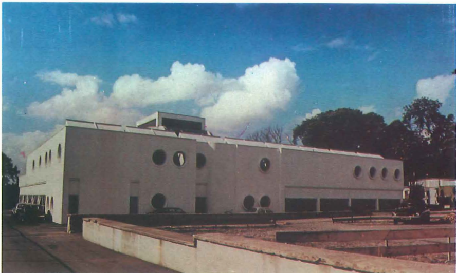
This modern exchange building at Roslevin in County Athlone houses Ireland's first digital exchange.
