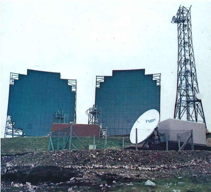
These dishes at Mormond Hill in Scotland communicate over the horizon with oil and gas production platforms.
