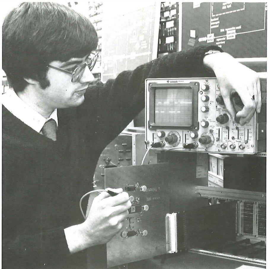
Author Gregory Coombs uses an oscilloscope to monitor the data signals on the supervisory system.
