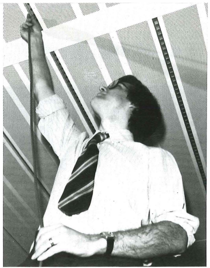
Guildford assistant executive engineer Alan Austin (left) checks the pressure drop across the adjustable air delivery slots using a manometer with the help of clerk of works technical officer Peter Woodward.
