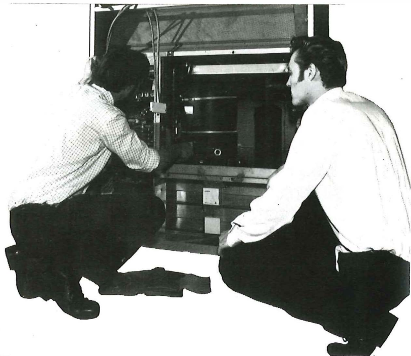
Above: The 15kW refrigeration section can be completely removed and replaced but can also be totally accessed for servicing or replacing components. Here, Peter Kiff (right) executive engineer in BTHQ's Building Services Division, and Alan Austin check over the refrigeration unit.
