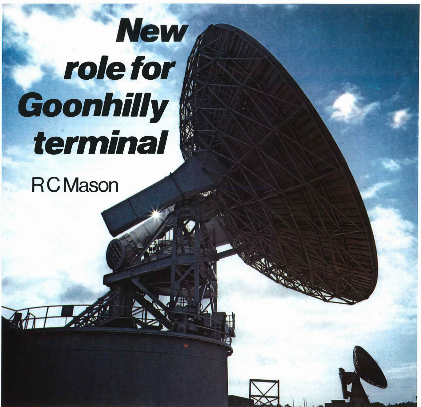
The Goonhilly IV terminal showing the beam waveguide.
