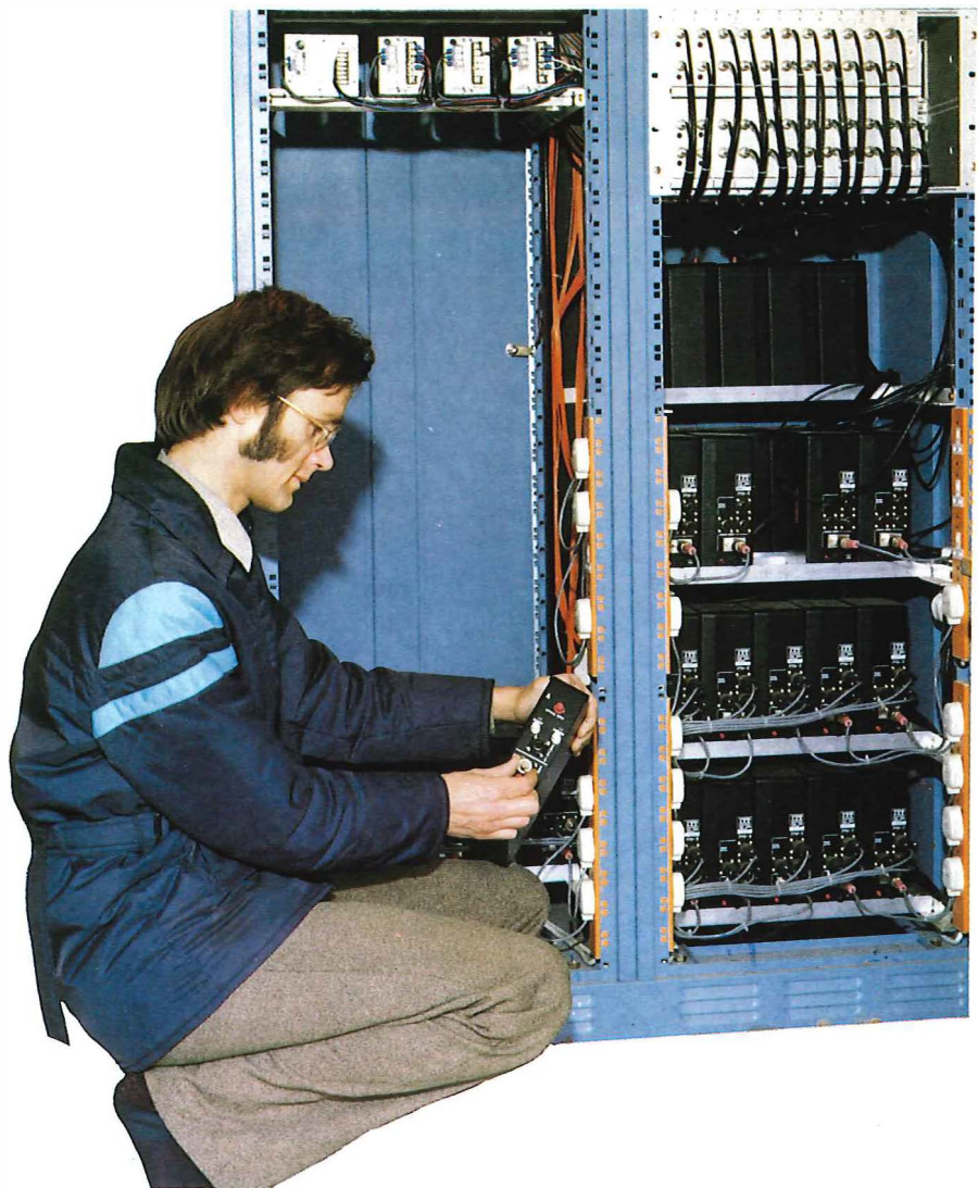
Dr J R Fox, author of this article, installs an optical receiver unit into the equipment rack inside the flexibility point of the Fibrevision system.
