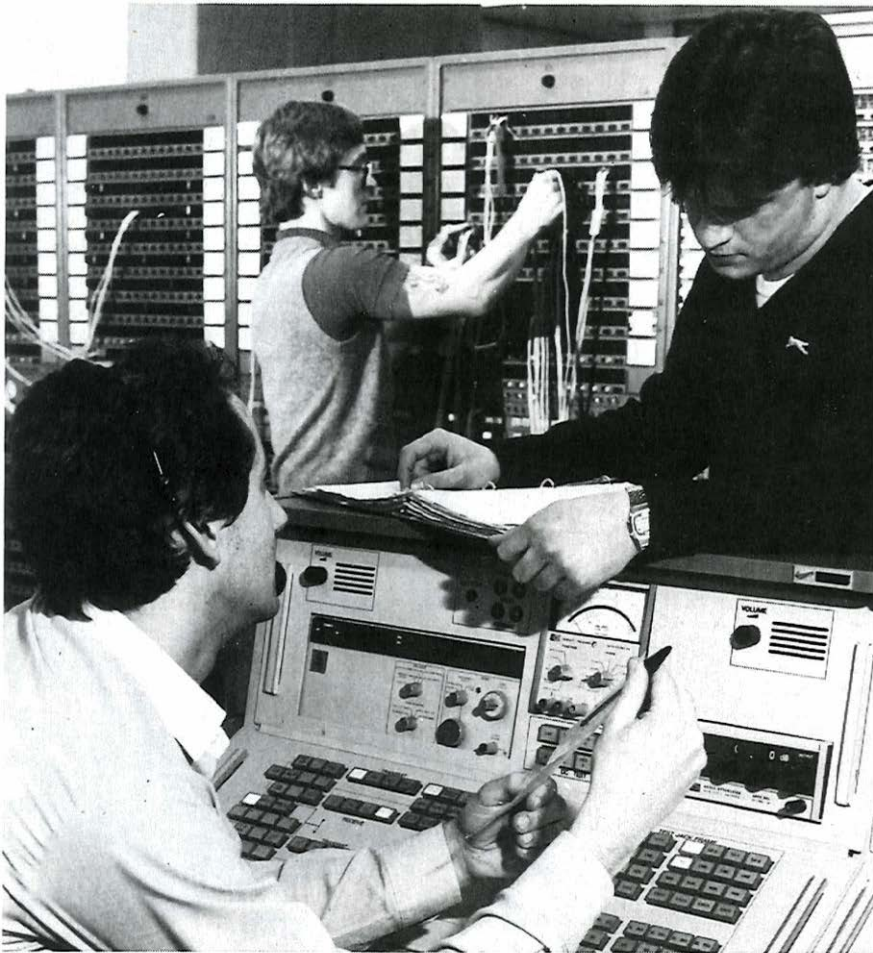
Technician Neal Oxley (seated) tests an international leased circuit routed to Sao Paulo, Brazil from the international maintenance centre in London's Mondial House while Roger Deller (right), checks a circuit routing document. In the background, technician Mervyn Bronze patches another circuit to the test console ready for checking.
