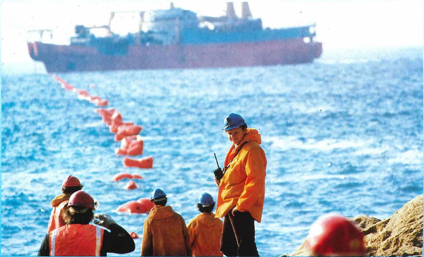
The shore end of the TAT-7 cable system is brought ashore at Porthcurno near Lands End.
