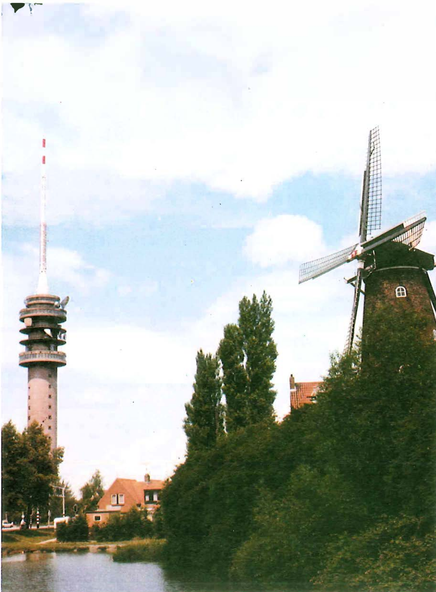
A blend of the new and the traditional . . . this telecommunications tower at Goes in Zeeland carries telephone calls and is used as a microwave link for broadcasting and television transmissions.
