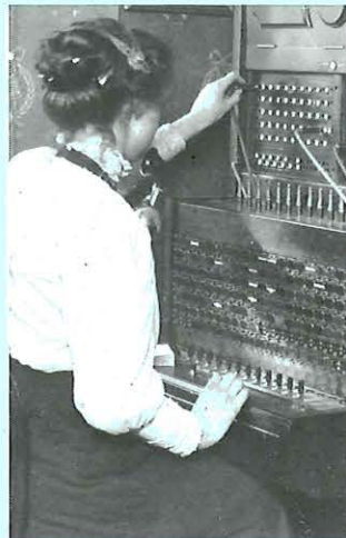
How it used to be – a busy switchboard 70 years ago.
