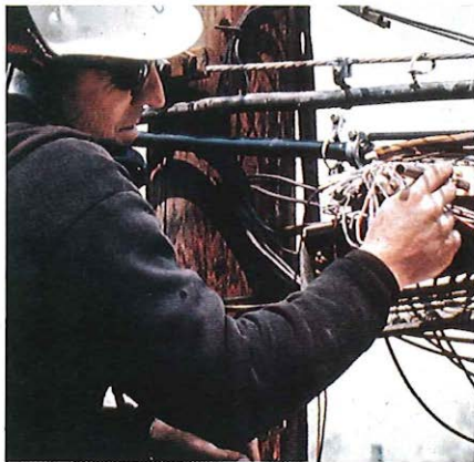
An Illinois Bell Telephone Company engineer checks out an aerial cable.
