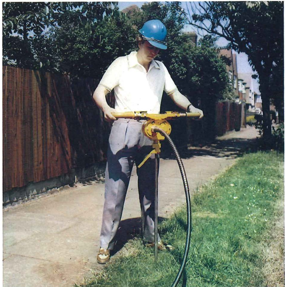
New equipment like this discriminatory borer is constantly being evaluated. It can penetrate the soil and reach duct or cable without damaging the service.
