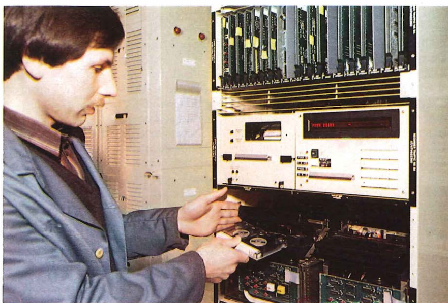
Technical officer Malcolm Walker removes a cartridge from the traffic recorder at Great Dunmow exchange, Essex . . .
