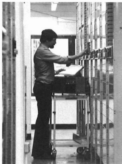
Below: Dave Dix, a technical officer, tests exchange line access in the Nat West building.
