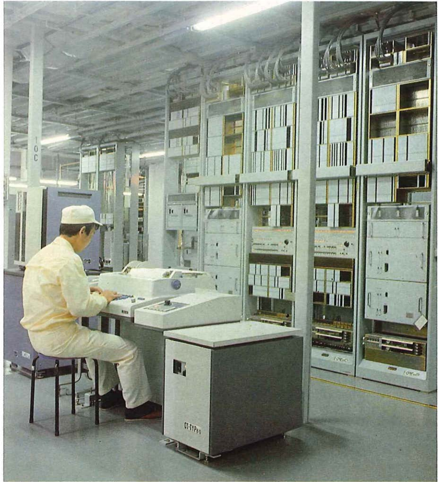
Japan has an extensive programme for introducing electronic switching. This is the D-10 electronic switching system.
