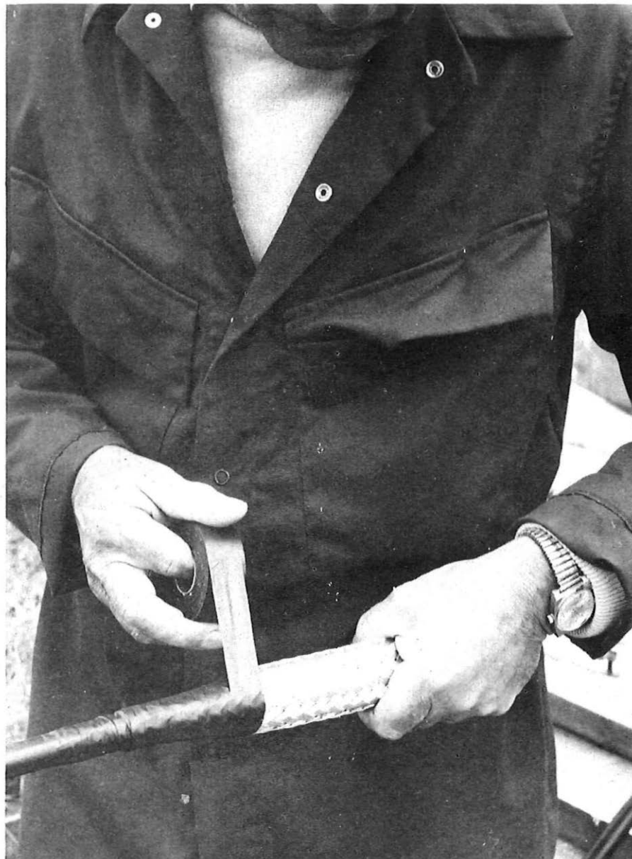
Technical officer Fred Honour tapes over the mild steel tubular mesh on a one-to-one cable before application of the shrinkdown sleeve.
