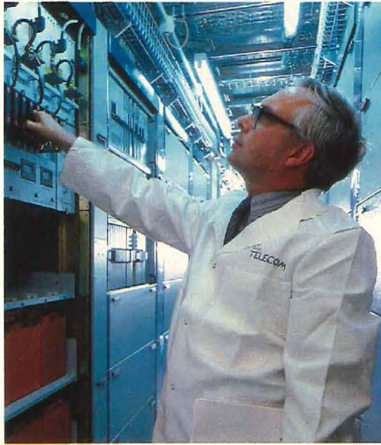
Right: planners need to consider the capacity of existing plant (like this System X exchange) while forecasting future traffic levels.
