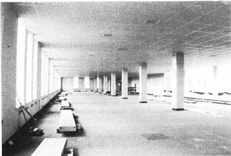
False floor and ventilated ceiling fitted
