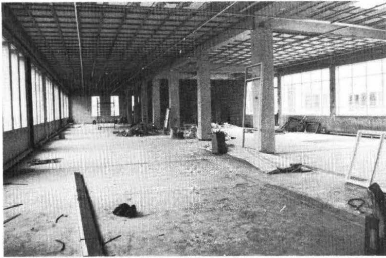
Refurbishment under way
