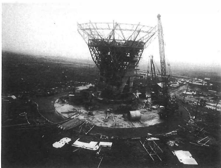
Figure 4 Aerial 1 under construction, March 1962
