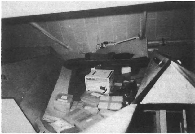
Fig. 6—Diverter A6A in operation
