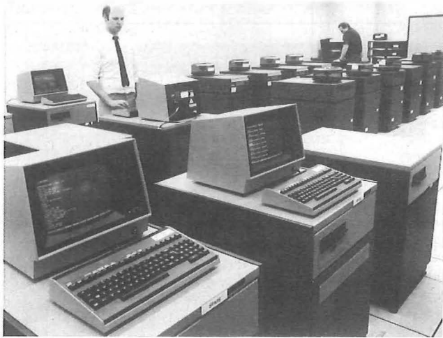
Fig. 5—General view of the computer room
