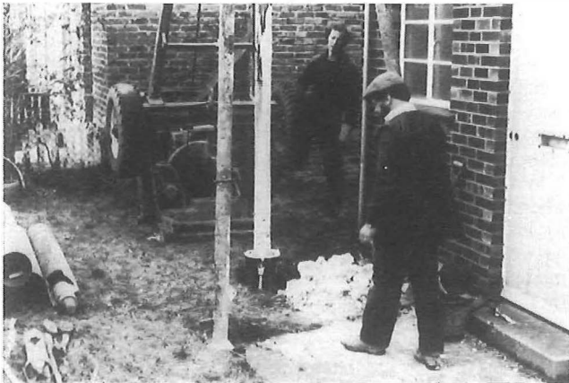
(b) Drilling boreholes
