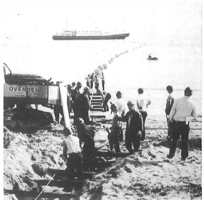
Fig. 12—CS D.G. Bast laying shore end at Broadstairs
