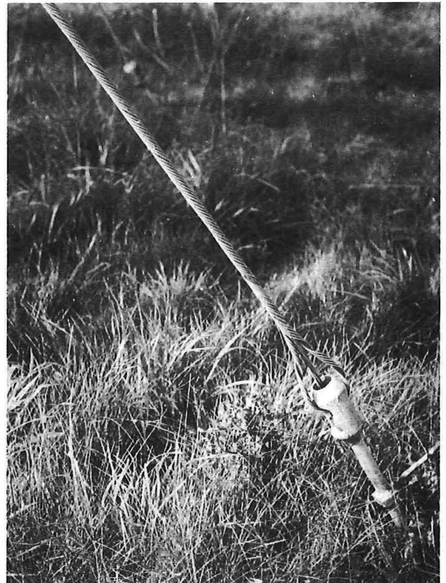
(b) Stay-grip terminating a stay-wire on a screw-type stay-anchor
