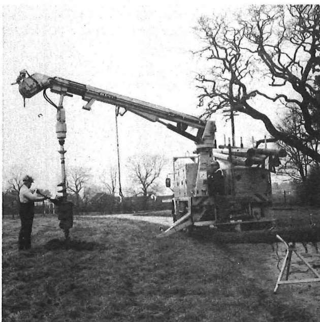
(b) Augering pole hole
