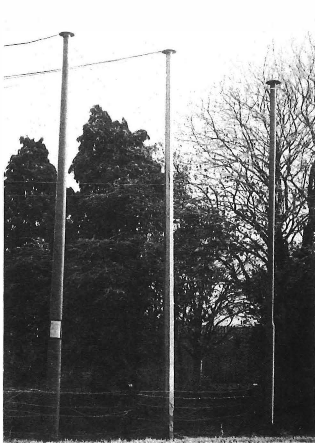
Left to right: GRP, sheet steel and two-diameter steel tube types
