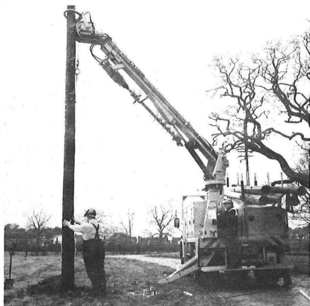
(a) Placing pole in position
