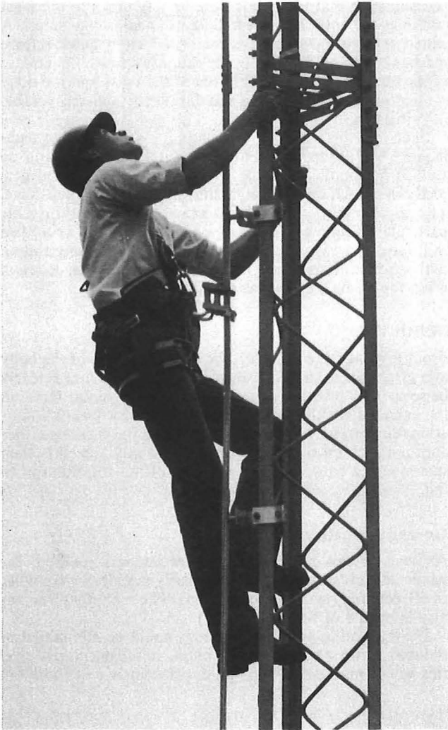
FIG. 2—Type 1 fall arrestor in use
