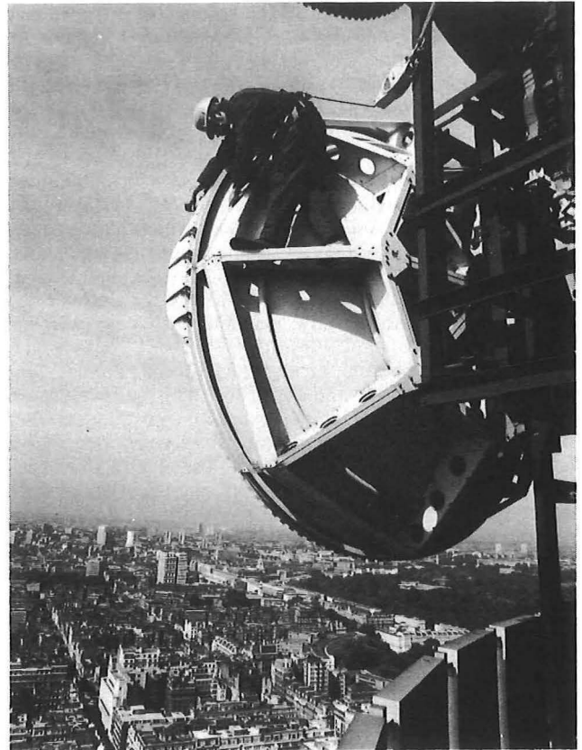
FIG. 3—Type 2 fall arrestor in use
