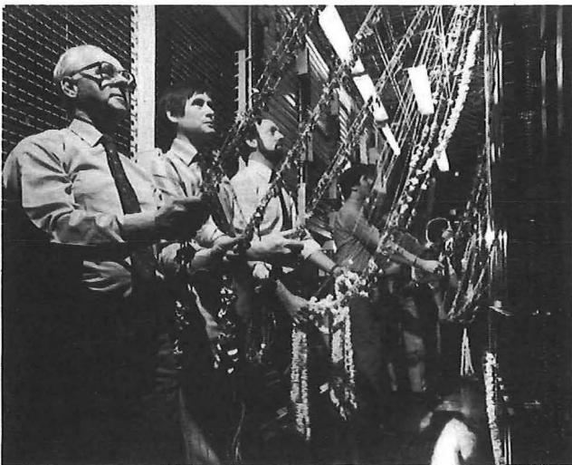
'Pulling the wedges' at Deal, in Kent, when the former Strowger telephone exchange was changed over to an electronic TXE4
