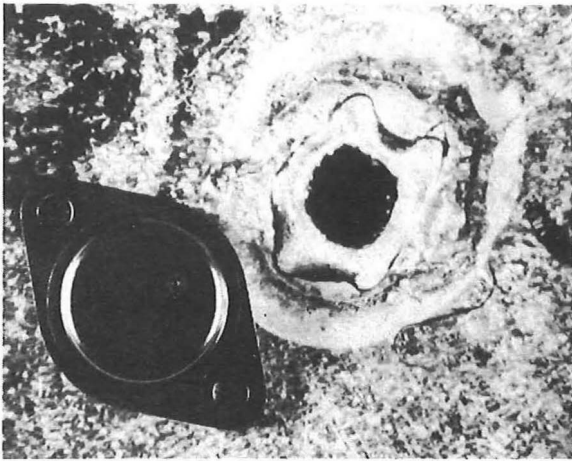
FIG. 2—A hole in the package caused by internal arcing between the emitter post and the metal lid
