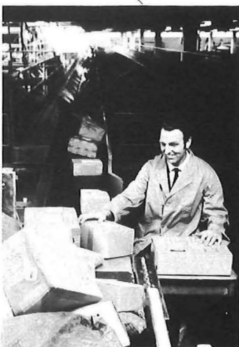
FIG. 25—A tilted-belt parcel-sorting machine seen from the operator's position
