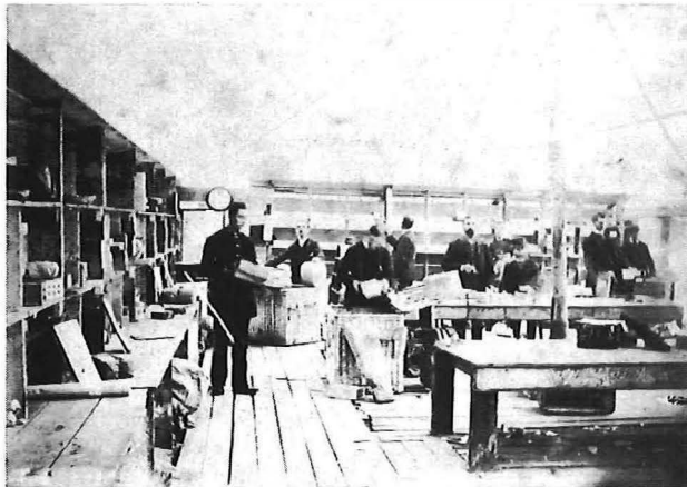
FIG. 9—The marquee erected at Glasgow to house the parcel-sorting operation
