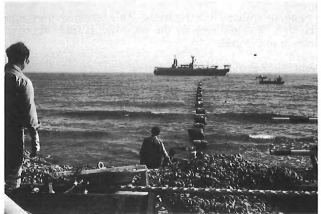
FIG. 4— CS IRIS laying the Drains Bay shore-end cable
