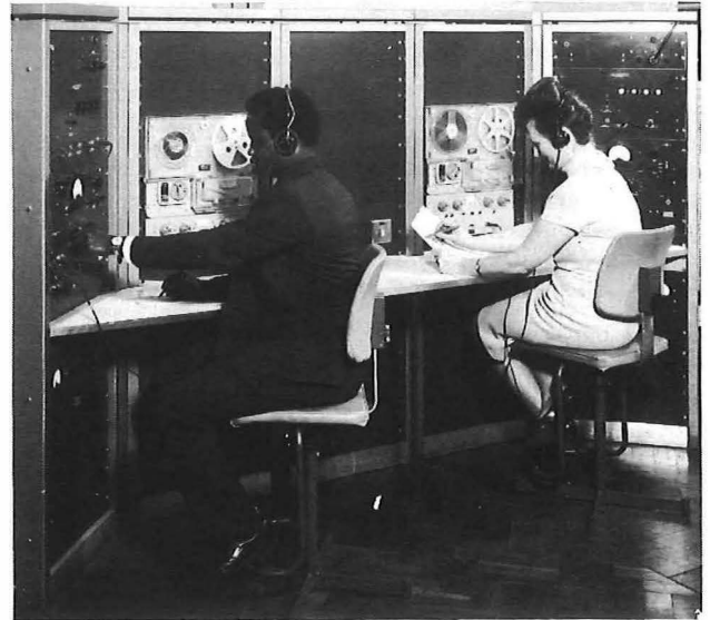
FIG. 6—Two rack-mounted SV5Bs
