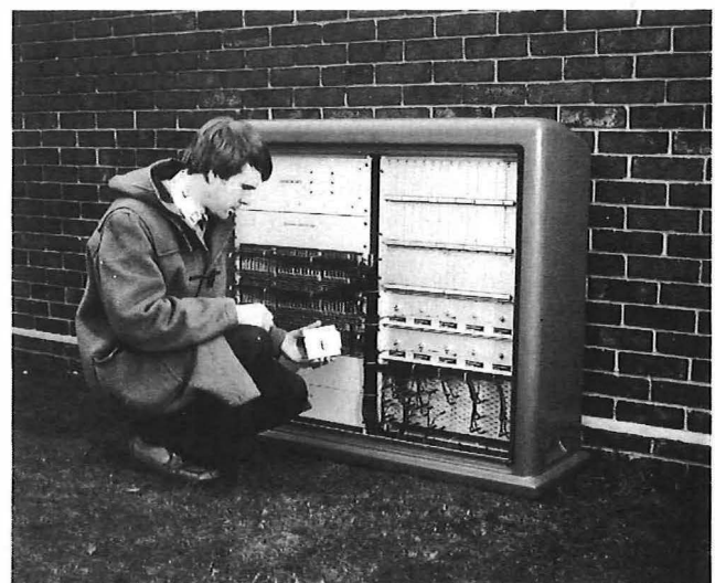
FIG. 5—Wideband switch point
