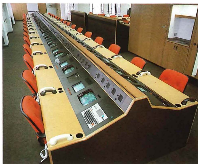
FIG. 1—City Business System installed at Godsell and Co. Ltd., London
