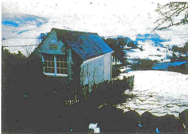
Building housing an early UXD5 installation in the Scottish Highlands
